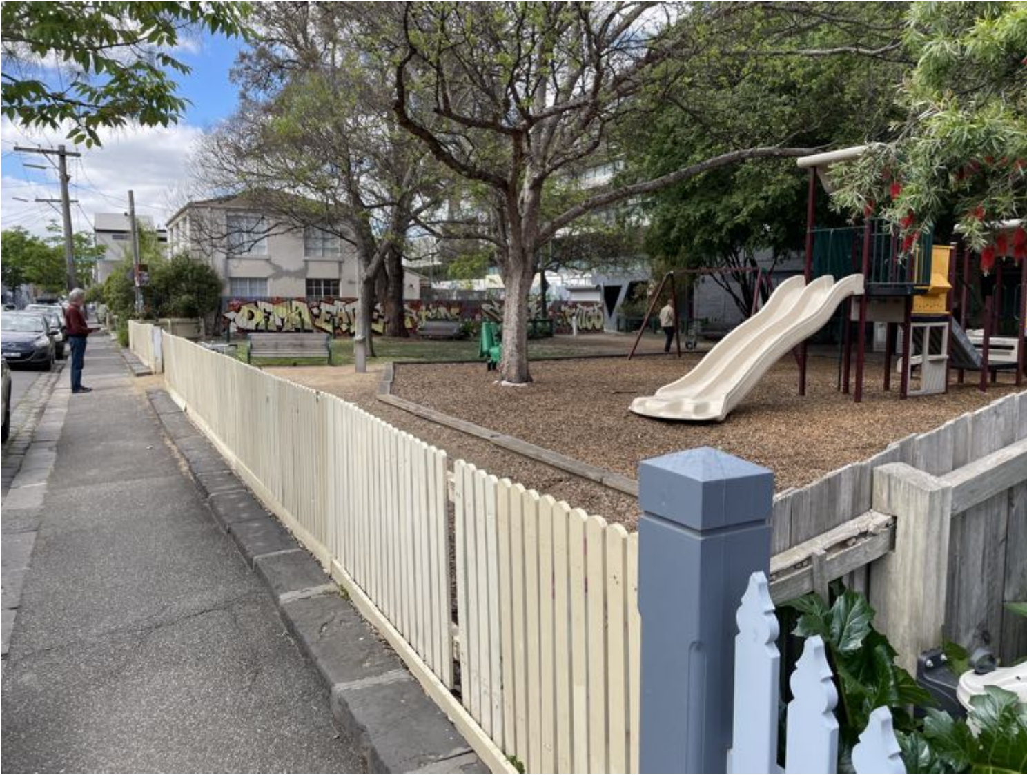
The northern boundary (Leicester St) with biege timber picket fence & bluestone kerb
