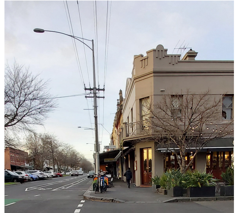
Footpath extension Rathdowne Street and Curtain Street
