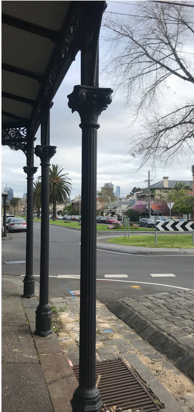
Heritage footpath canopy Canning Street at Pigdon Street
