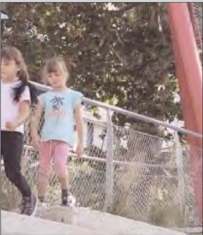
STEEL AND TENSILE MESH BALUSTRADE
