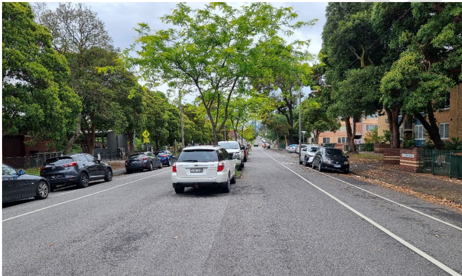
Figure 2-3: Wilson Street, looking south from Park Street
