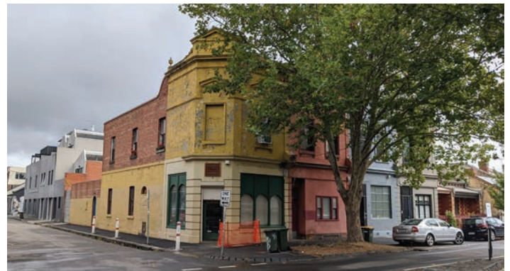
Contributory dwellings along Westgarth and Fitzroy Streets
