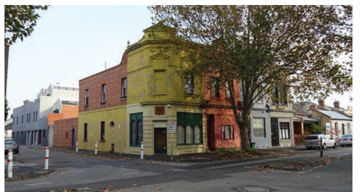
Corner profile of Westgarth and Fitzroy Street
